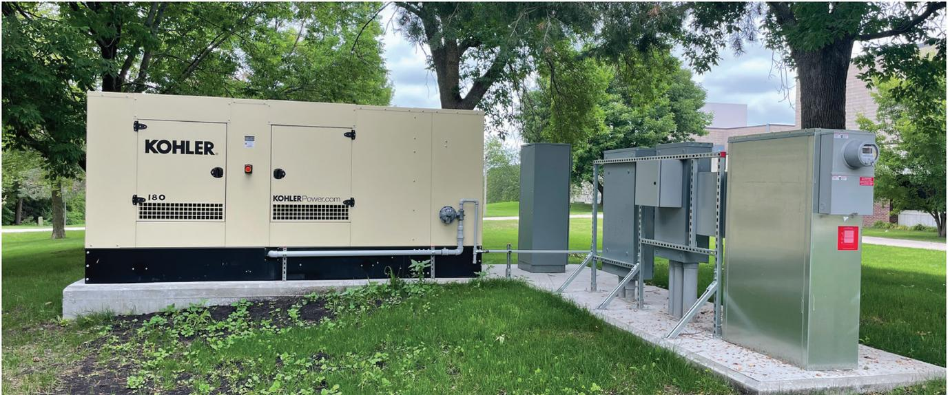
A KOHLER® 180REZXB generator set and KCS-DMTA-0400S and KCS-DMTA-0200S transfer switches at North Iowa Community College
