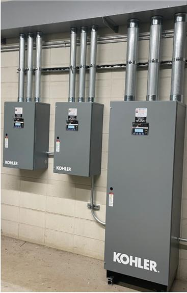
Kohler KCS-DMTA-0104, KCS-AMTA-0104 and KCS-DMTA-0400S transfer switches provide smooth transitions for the microgrid system
